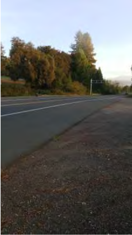
The crossing at highway 101 was completely removed
