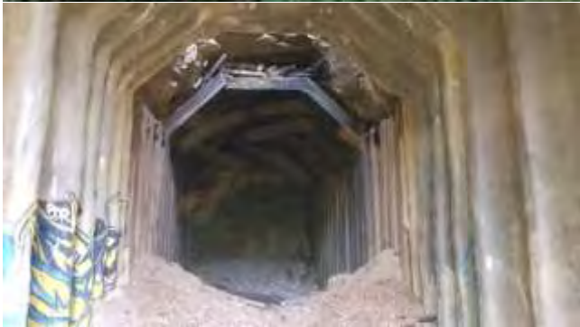
North end of the tunnel
