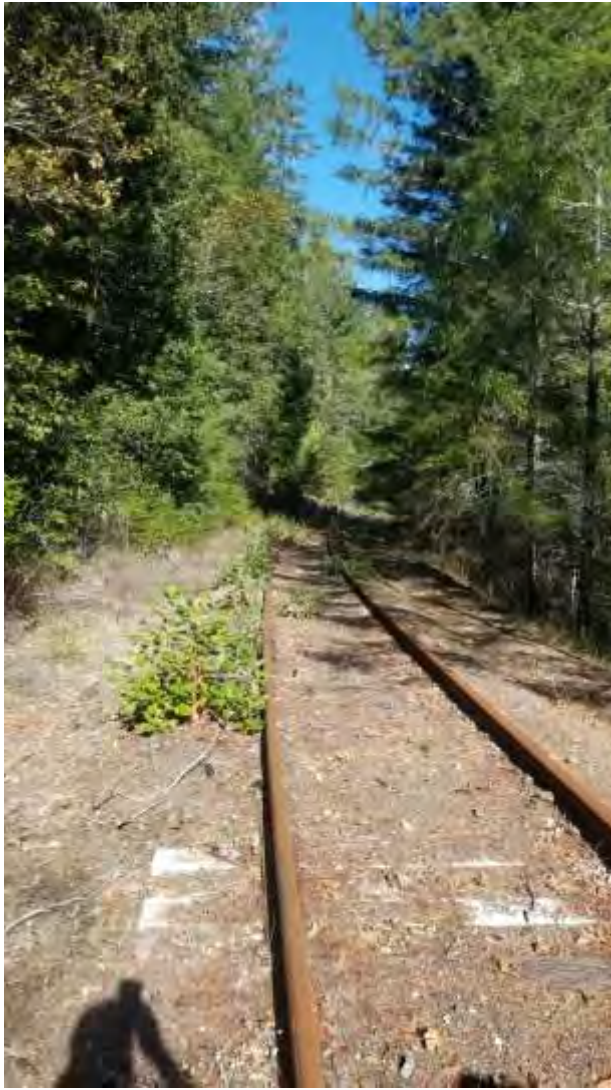
MP 147 131 pound rail, Tie condition good vegetation good,
