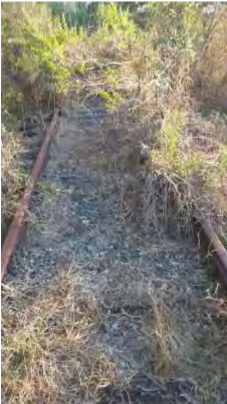
MP 141.5. Vegetation: Poor Ties: Good
