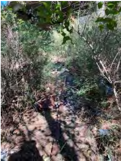
Milepost 149.5, vegetation condition extremely poor. 110 lb rail in good condition, tie condition poor
