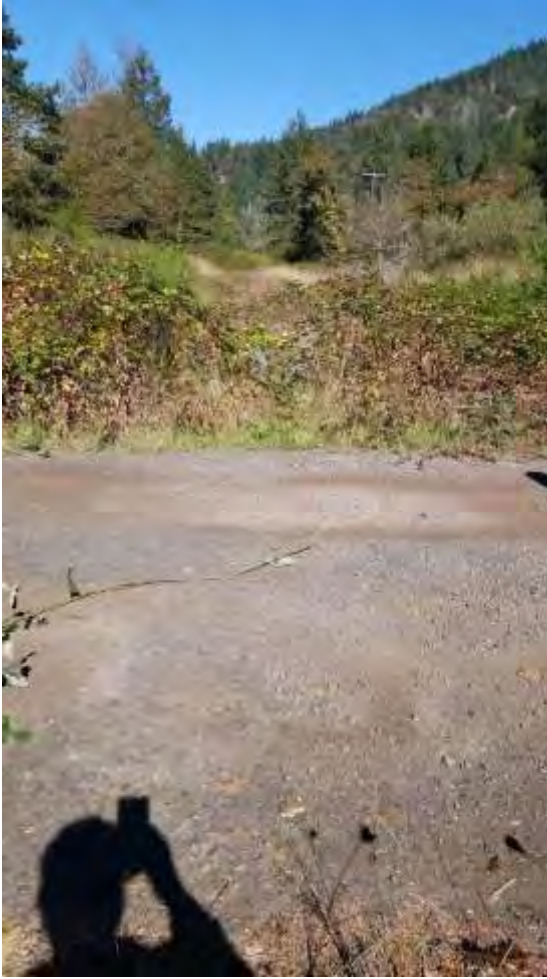
MP 150, private crossing, 112 lb. rail in good shape tie condition poor, vegetation extremely overgrown.
