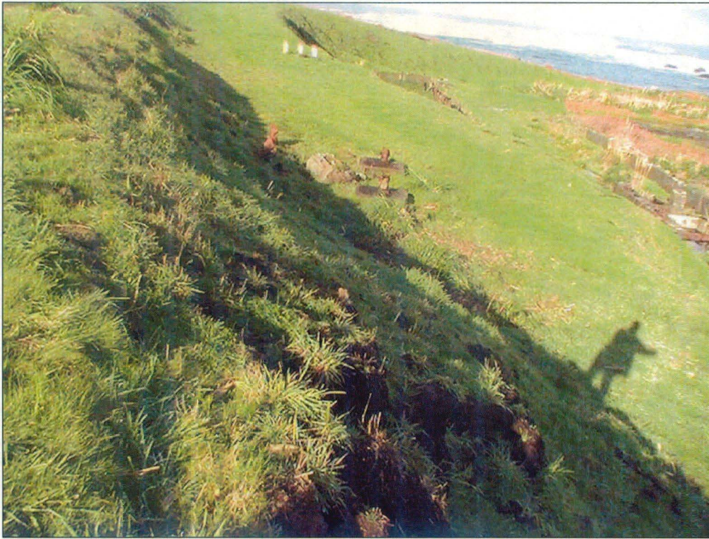
View of the north wall looking towards west, showing surficial sloughing
