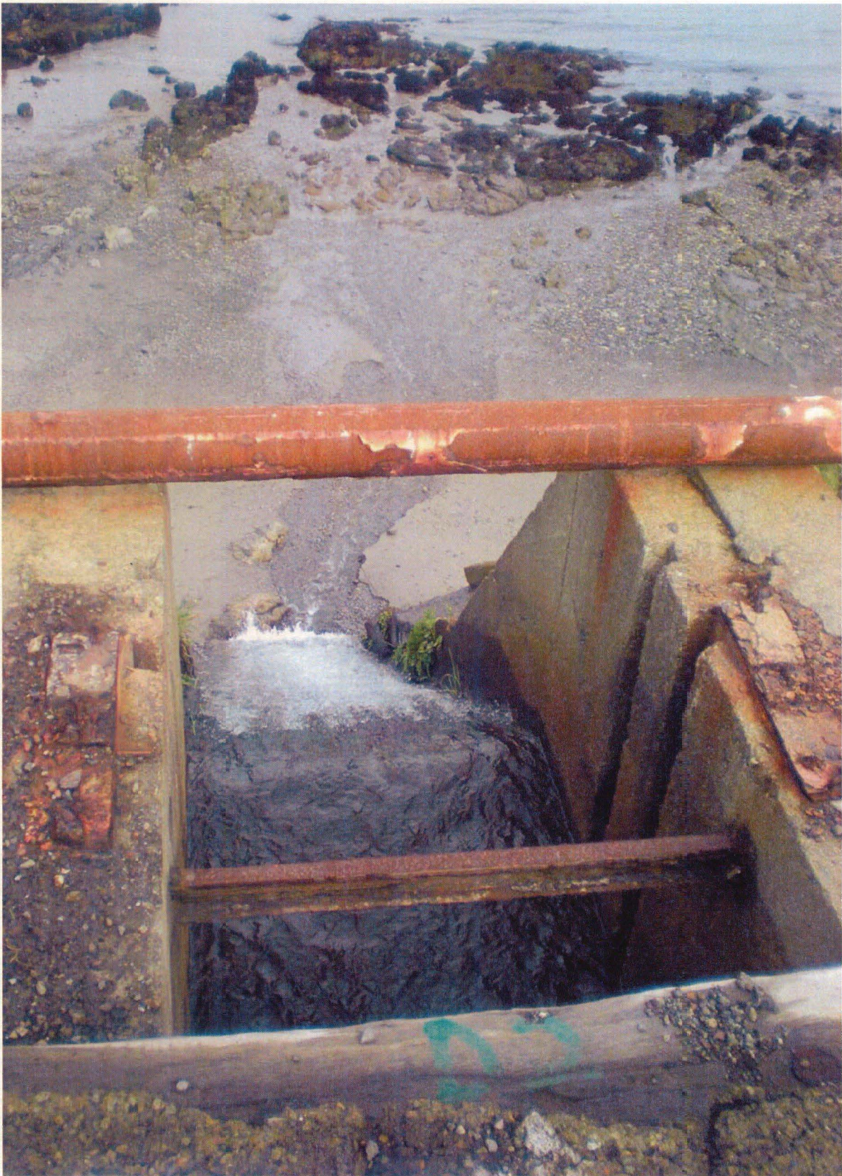
View of the spillway discharging directly on to the beach
