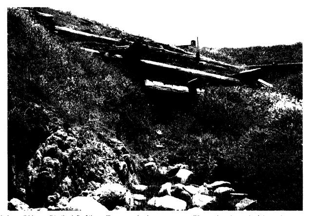
The timber-cribbing wall to the left of the spillway remains in very poor condition and continues to deteriorate Embankment material continues to be transported from behind the wall, opening voids and causing a loss of contact and support between the structural timbers and the supported embankment.
