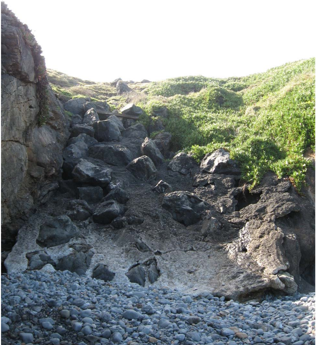
Photo: Rip-rap and concrete closure of the historical stream channel from the South Ponds area. The outlet is a small beach area adjacent to Soldier Bay.
